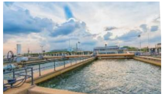
Water treatment plant use filtration and other methods to purify groundwater or surface water.
